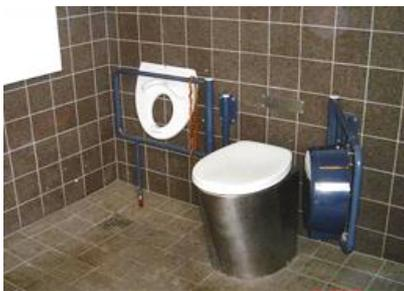
The toilets were built with stainless steel stools connected to Clivus Multrum units placed in the basement.
