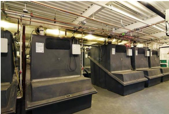
The Eco-Restroom accommodates more than 1/2 million visitors per year. The 15 foam-flush toilets use only 6oz. of water per use, resulting in a savings of more than one million gallons of water each year, as compared to conventional low-flow (1.6gpf) toilets.
